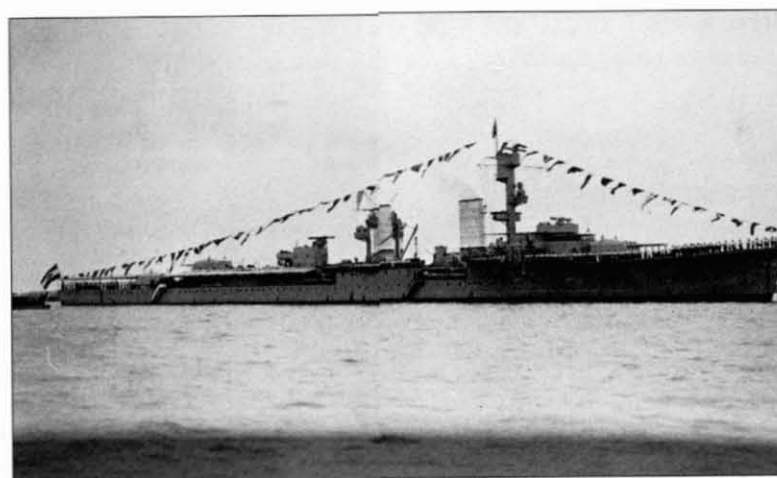
Light cruiser Nürnberg . German designers have helped historians by including a well for torpedo tubes somewhere near the forward funnel. In this case the black box-like feature can be seen between funnel and bridge.
