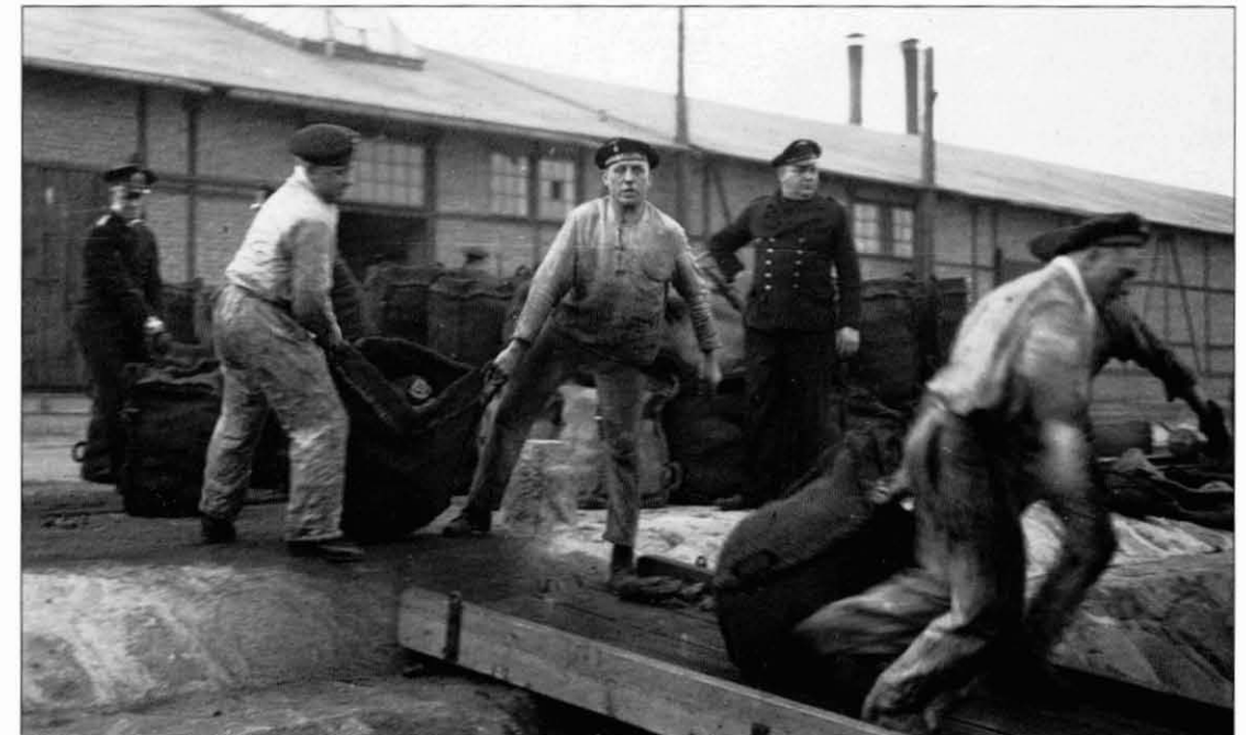
After the First World War the majority of minesweepers were converted to burn oil instead of coal, but shortages meant they were changed back again for the Second World War. This shows coal sacks being brought aboard a minesweeper.
