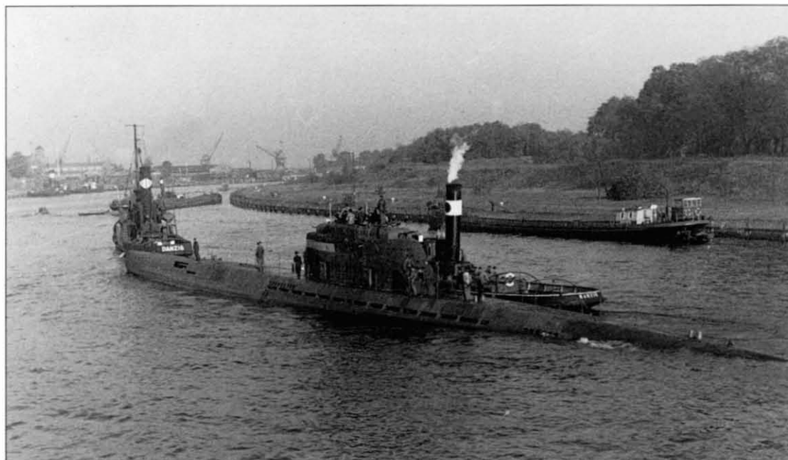
One of the new large electro-boats of Type XXI in Danzig towards the end of the war. It was planned that these should replace Type VII as the mainstay in the Battle of the Atlantic, but only a handful were ready by the time the war started.
