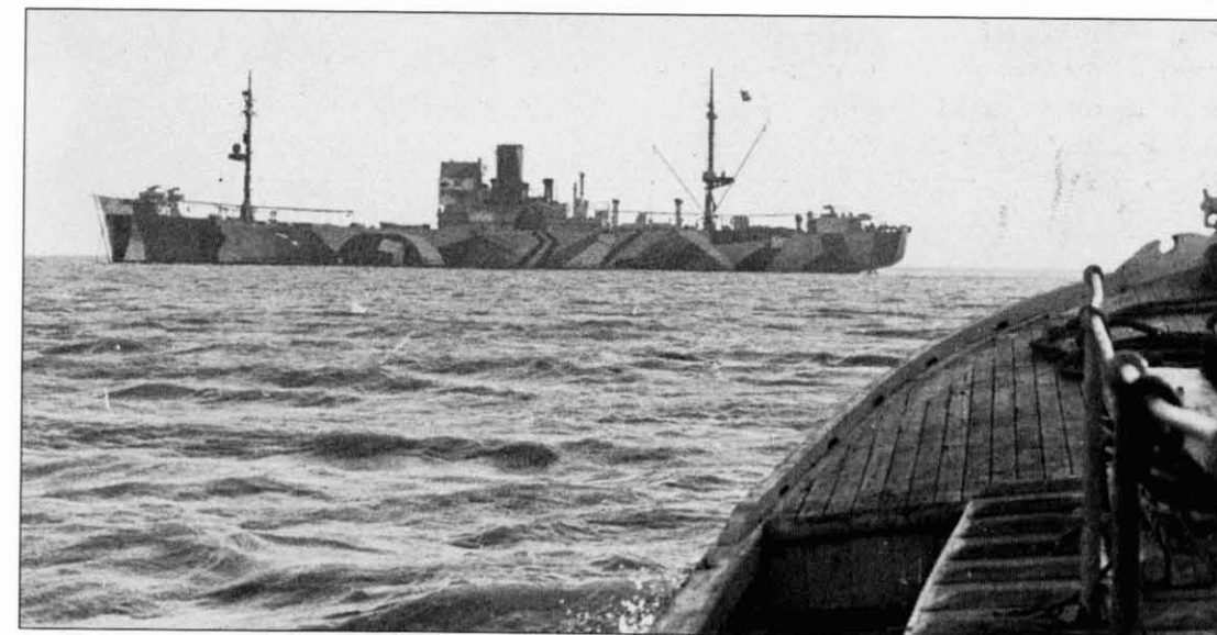
A Sperrbrecher or barrier breaker lying at anchor. These ships were filled with flotation aids so that they could sail in front of others to detonate mines. Life aboard them must have been somewhat uncomfortable, despite living quarters having been provided with extra insulation.
