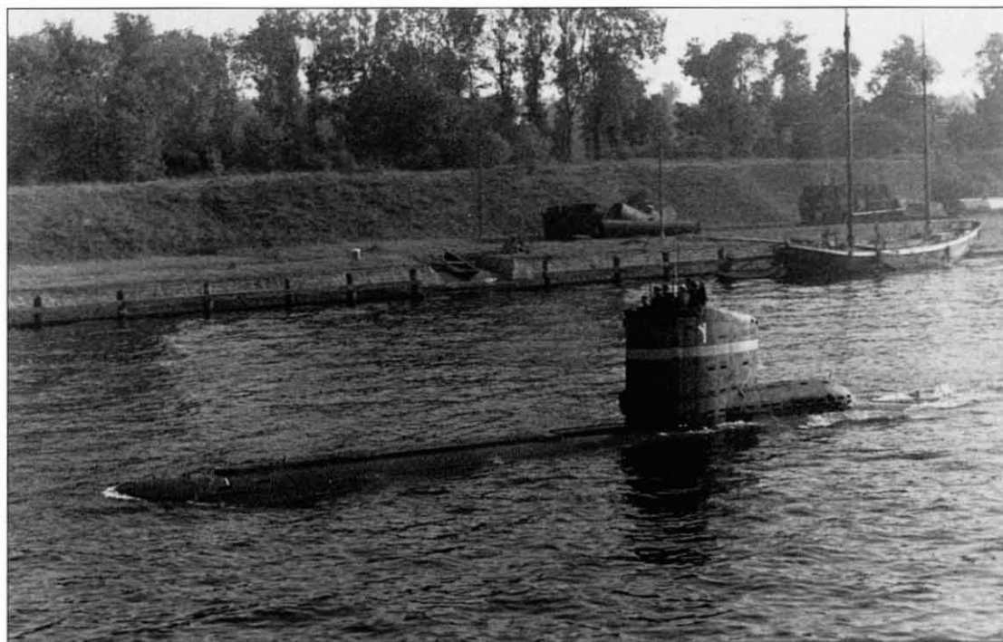
Type XXIII, a small electro-boat, towards the end of the war. The inside was so cramped that torpedoes had to be loaded into the tubes from the outside and there was no room to carry spares.
